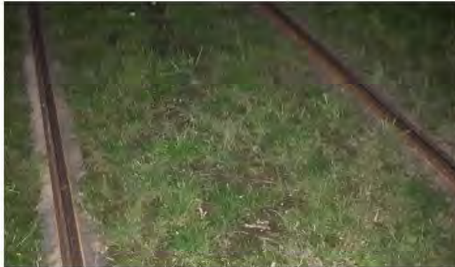
Figure 7. Embedded track in Uithof line.
